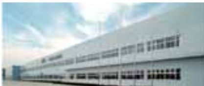
Fujitsu General Central Air-conditioner (Wuxi) Co., Ltd.
