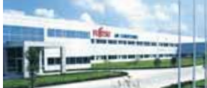
Fujitsu General (Shanghai) Co., Ltd.
